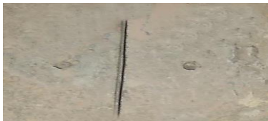
Fig.1. Horizontal discharge slot
