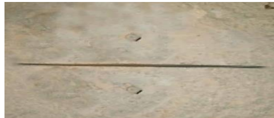
Fig. 2. Vertical discharge slot
